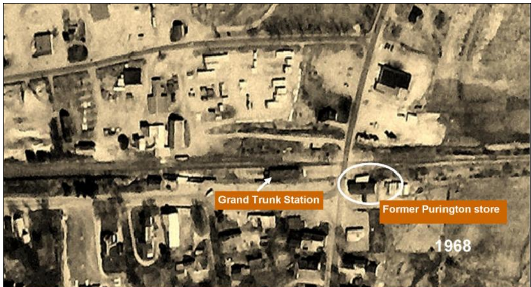
1968 aerial photo shows the rail siding where Woodbury & Purington shipments were loaded and unloaded. Later heating oil was delivered here by rail for Irving L Carver Co.
