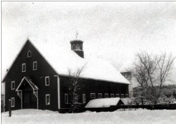
A.S. Bean's 50 by 125 foot barn built in 1890. It faced Route 2 approximately opposite the rail depot.
