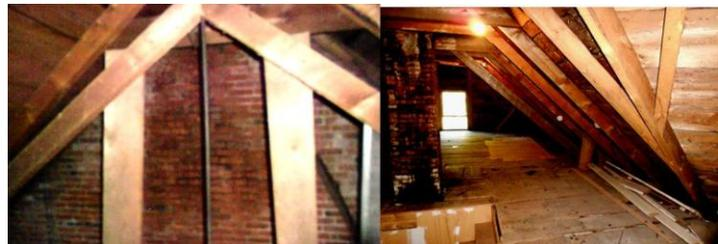
Roof connects directly to the brick building's wall, left and main roof interior, right
