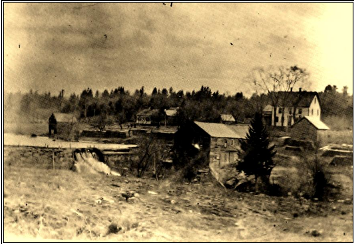
Above: photo shows the completed large upper dam on Mill Brook. To the right of the gates/slucie way is the large building - the former Clough mill which had housed the corn canning factory (1880-1890) and was converted by Hodsdon to manufacture lumber. Bethel Historical Society photo.
